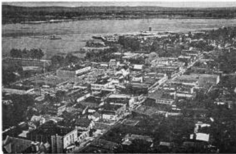
AERIAL VIEW OF PEMBROKE
